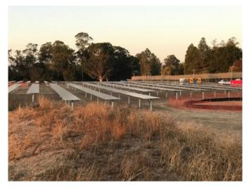
Figure 9 - Typical Sun Tracking Photovoltaic Array at DSH-Napa
